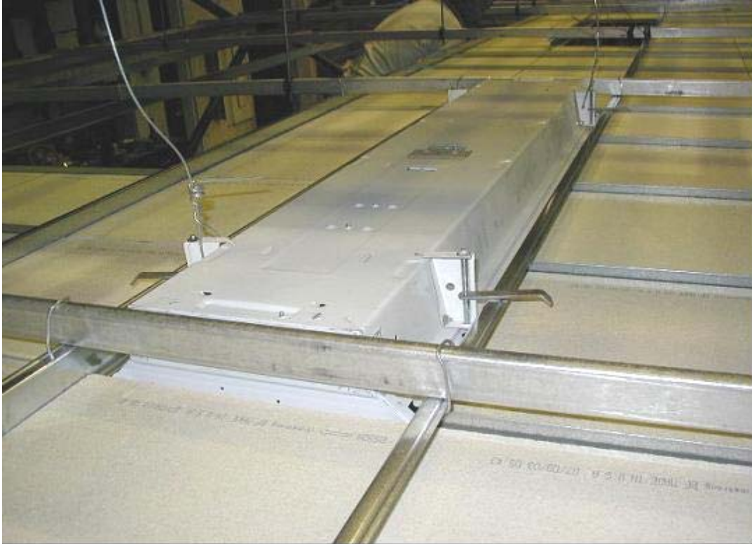
Figure 2–28. 12 in. by 48 in. (0.30 m by 1.22 m) fixture with safety clip and wires in ceiling system CS1.
